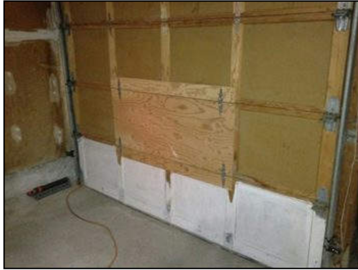
6. Repairs to garage door
