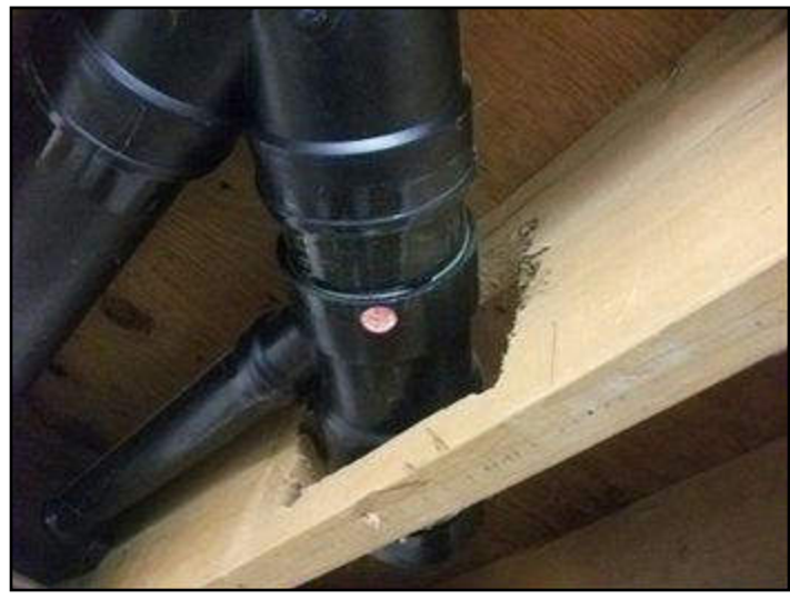
8. Joist damaged
